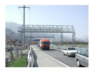
Furthermore, the Customs Administration checks that the HVC declaration is correct with fixed and mobile monitoring points in traffic. The data from the recording device is transmitted via the DSRC radio link by the current 27 fixed monitoring installations on the Swiss motorway network and is automatically compared with the data (number plate, vehicle length, etc.) captured electronically by the installation.
